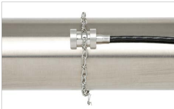
PT100 transducer fixed to pipe
